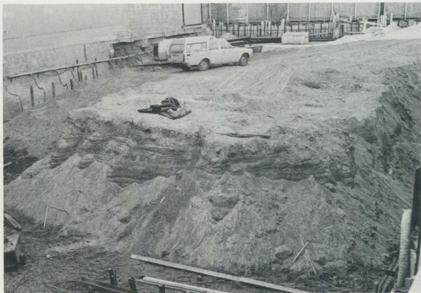
Fig. 35. Skärning i älvsediment. Stadsdelen Öster i Jönköping. Section in fluvial sediments. From the Öster district, Jönköping city.
