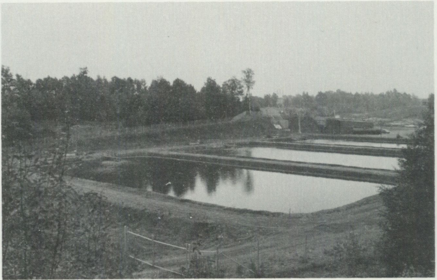
Fig. 15. Dammarna för utfällning av järnföreningar i Malma grustag (2j/3j). Foto förf. 1982. Three basins in the gravel pit north of Malma (2j/3j) in which iron compounds precipitate from the natural and artificial ground water pumped up at Fågelbacken, situated between the infiltration place in Fig. 14 and these basins.
