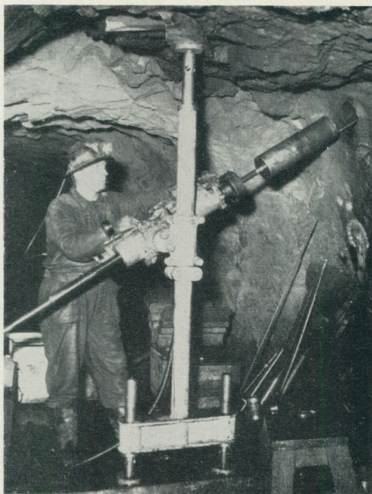
Fig. 8. The diamond drilling apparatus now exclusively used.
