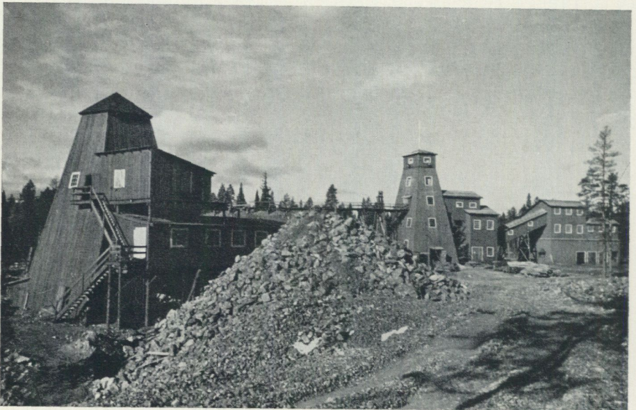
Fig. 2. The Lainijaur Mine at the closing down in 1945.
