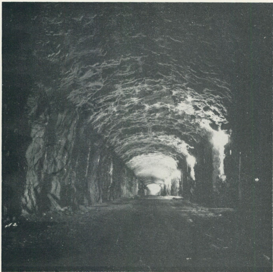
Fig. 3. Interior of the outlet tunnel of the Parteboda power plant (width about 10 m, maximum height about 9 m, area of cross section about 85 m 2 ). Photo from N. E. by P.H. Lundegårdh in 1960. ©
