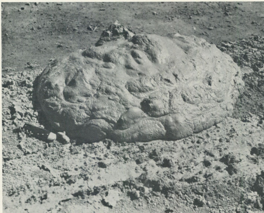
Fig. 46. Frost boil on a road in Indal, Medelpad. Notice the knife as a scale! — From G. Lundqvist (1959 a, Fig. 50). Photo by Th. Lundqvist 1957.
