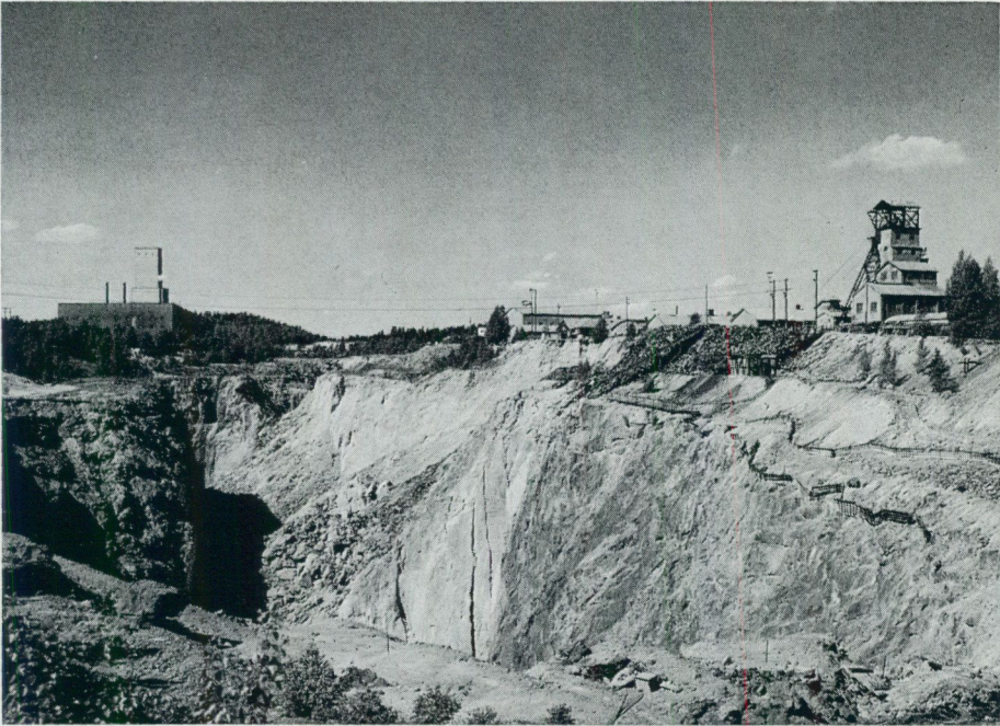
Fig. 18. The Boliden open pit. The central shaft appears to the right and the dressing plant to the left. The subsidence around the great fault and its branch-line is seen in the centre of the picture. Photo in 1962.
