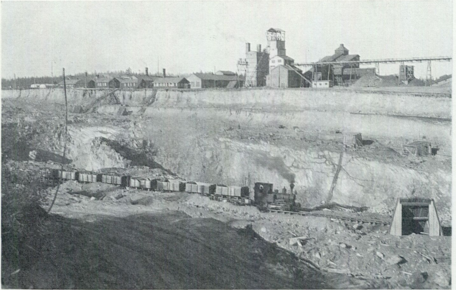
Fig. 3. Development of the open pit at Boliden. The overburden at the east end was more than 20 m thick. About one million cubic-metres were removed. Photo from 1934.
