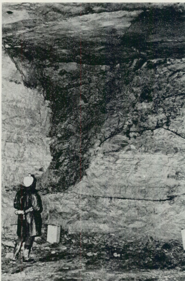
Fig. 4. Trattformad breccia i sandstensgruvan i Kvarntorp. Funnel-shaped breccia in the sandstone mine at Kvarntorp.
