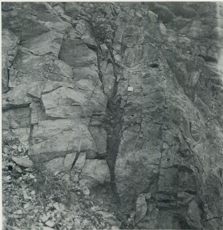
Fig. 9. Fissure with alum shales. The bedrock is strongly fractured (Table 1, no. 19).
