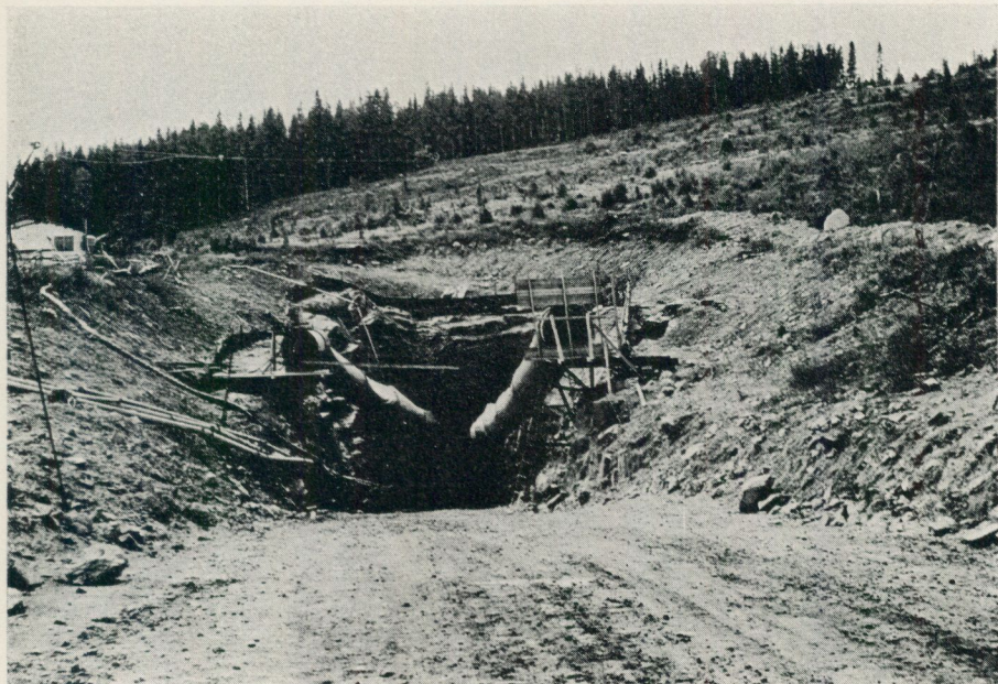
Fig. 2. Entrance to the tunnel near Alberget.
