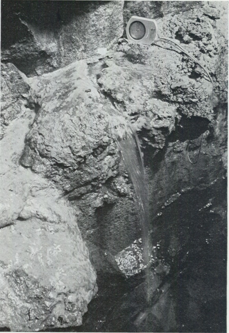
Fig. 13. Water inflow from an aperture in a horizontal fissure. Large quantities of iron and manganese sediments are to be found at the aperture. (Photograph by G. Hansson.)
