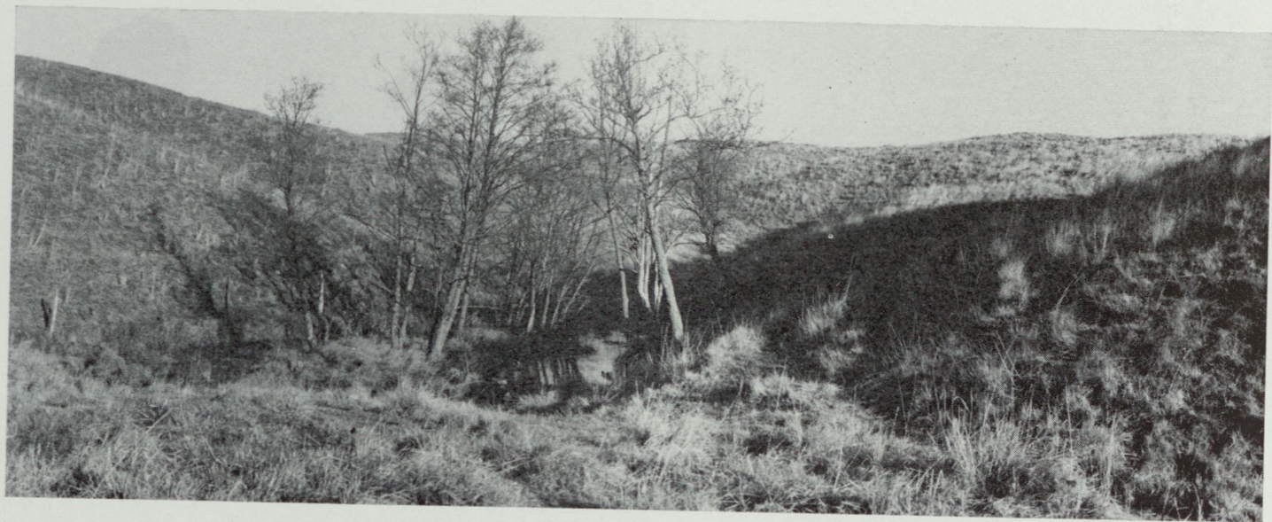
Fig. 15. A gully close to the western part of the Måssen landslide. It was dammed by the quick clay that flowed upstream the channel from the Måssen area and now forms a terrace bulge in front of the gully.
