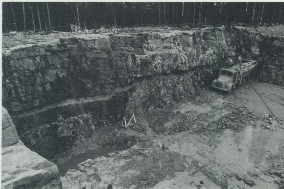
Fig. 10. View of the superficial rock mass with extremely wide apertures which are filled with a silty sediment. Photograph by G. Hansson/N.
