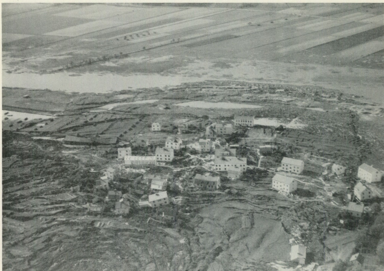
Fig. 20. Aerial photograph of the slide cavity seen from the east. The large slide element denoted as No. 5, in the north-eastern part of the slide cavity, is seen in the foreground, on the right. Those houses which are more or less inclined indicate the slide elements originating from the initial stage of the slide, which are visible behind the slide element No. 5. The valley flat was divided by the slide into two broad slide elements, which are situated outside the above-mentioned portions of the slide cavity. These slide elements are still partly covered with water from the river. The wide bow-shaped group of slide elements caused by the rise of the river bottom is seen in the area adjacent to the river. (Photograph by F 9.) Godkänd av Försvarsstaben 11/3 1955.
