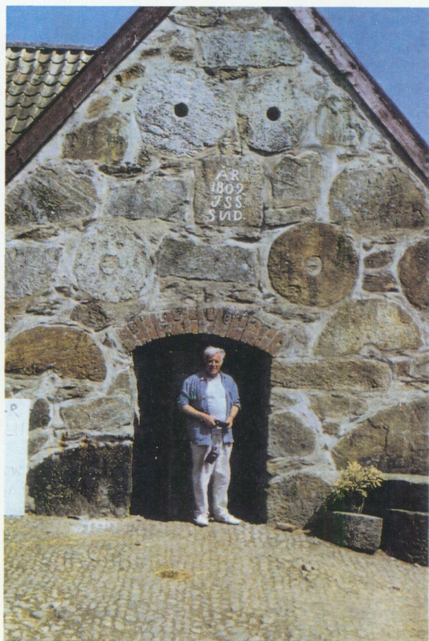
Fig. 35. The senior author at Vittseröd manor-house. Note the Höör Sandstone millstones in the wall. Near Locality B3. Photo: A. Ahlberg.
