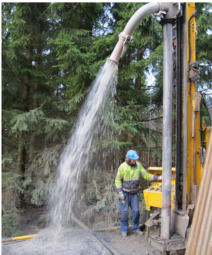
Figure 9. The drilling rig used for the drilling of wells is large and heavy. It is important for the contractor to take care in order to minimise any damage, especially on sensitive ground. It is also important to keep the equipment in good condition in order to prevent diesel or oil leakage.
