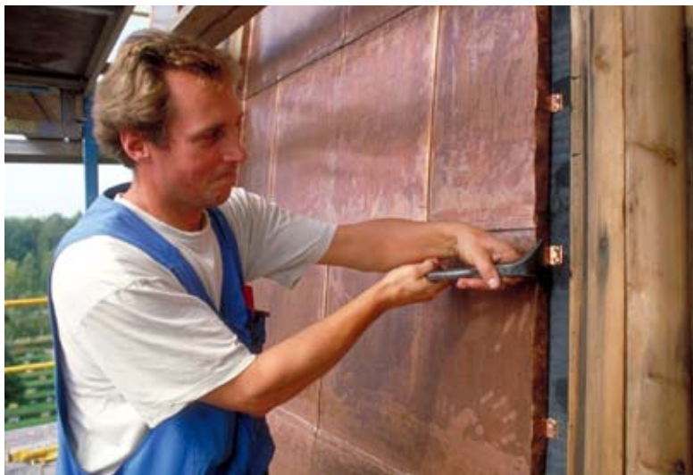
Copper sheeting on a church roof.
