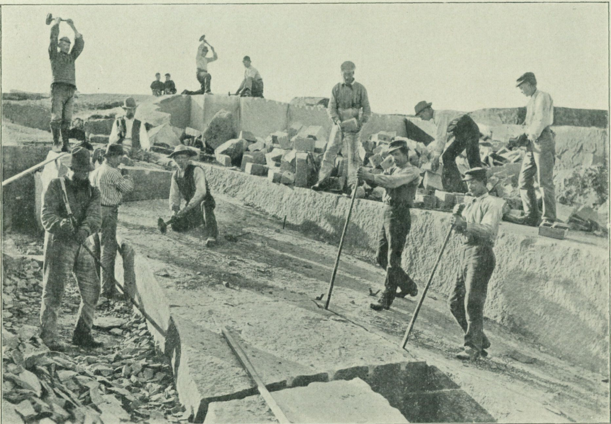
Bohuslän granite-quarry on Malmön off Lysekil, illustrating the marked joints of the granite.
