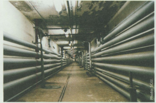
The underground oil storage facility in Jönköping, southern Sweden.
