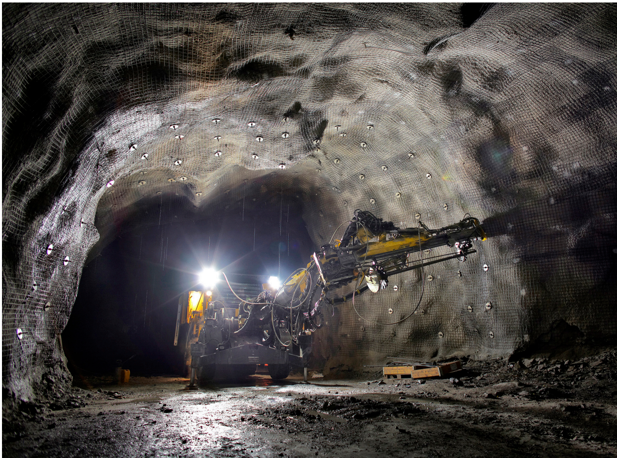
Rock reinforcement work. Photo: Fredric Alm/Alm & ME
