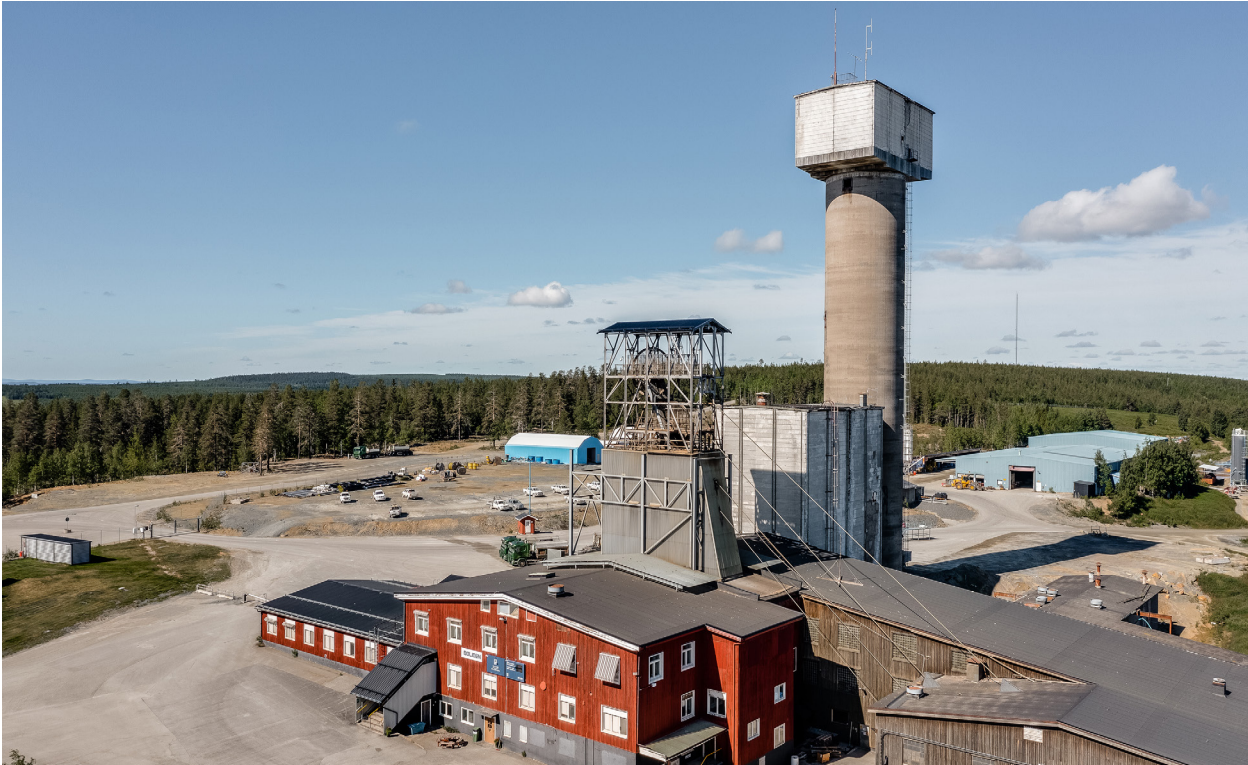
Kristineberg in the Boliden area. One of the applications for a mining concession granted in 2023 was Kristineberg K no. 1. Photo: Boliden
