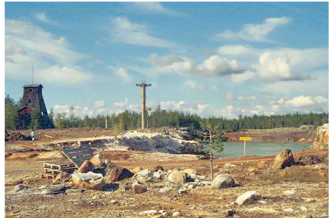
The Rakkejaur head frame and water filled open pit before the finishing treatment.
