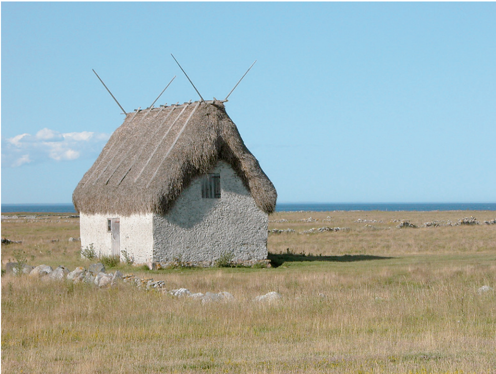
Old gutnian house with a roof of Cladium mariscus .
