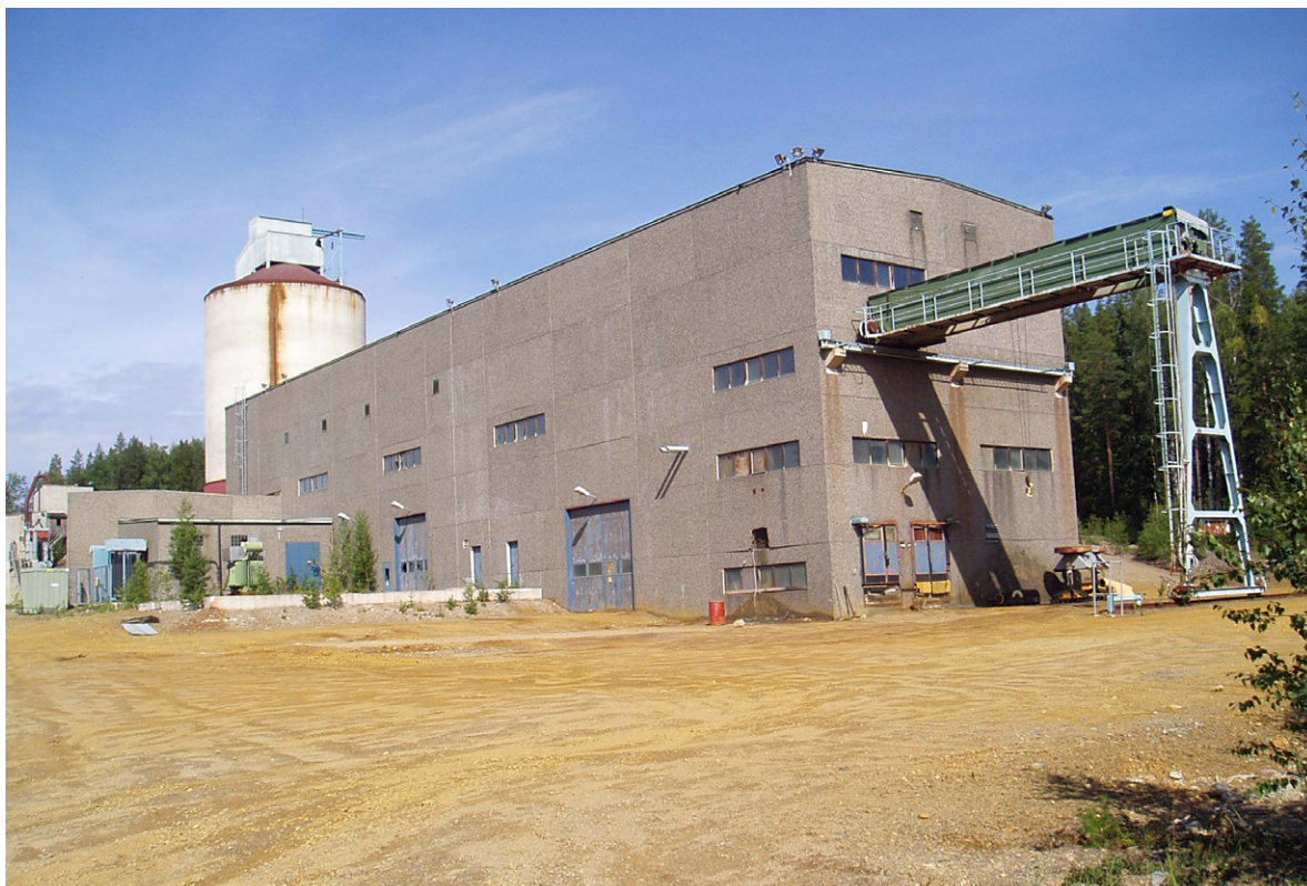
Fig. 13. Anrikningsverket vid Enåsens nedlagda guldgruva innan byggnaden monterades ner. Foto: Kjell Wallin. The dressing plant at Enåsen gold mine before the building was taken down and moved to Ljusdal.
