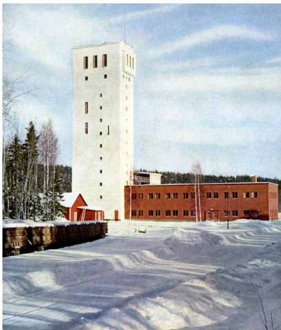
Fig. 31. Vingesbacke gruvlave 1956. Foto: ur boken Hofors Bruks historia. Vingesbacke head frame. Photograph from 1956, when ore production started.
