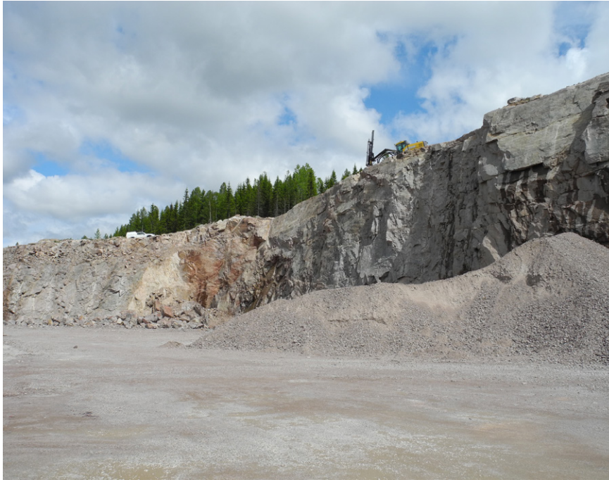
Mellanbergets krossbergs- täkt i granit. The aggregate rock quarry in granite at Mellanberget.
