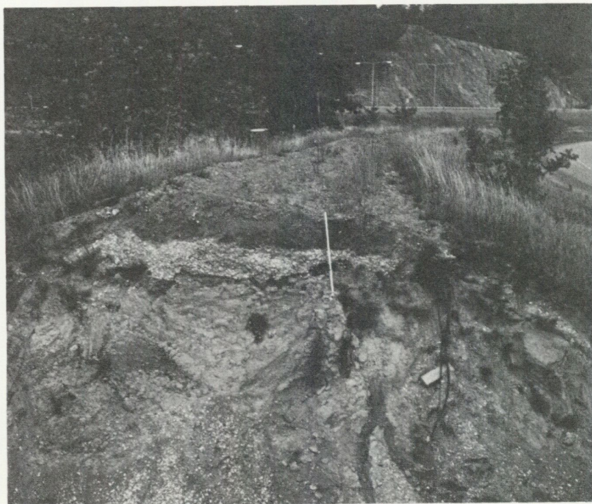
Fig. 6. Section of the former embankment of the state railway northwest of Uddevalla. The present highway and railway are seen in the background. The section shows the technique of railway construction in the Uddevalla area at the turn of the century. On a body of sandy-gravelly material (glacifluvial sediments and till), a 20–30 cm thick shell layer is visible below 30–40 cm of sand at the top. On the slopes there is clay 10–20 cm thick and covered by sand. The white stick where the right-hand rail used to lie is 1 m long. The railway embankment will be pulled down and the shells will be spread over again. — Photo CF 1976-09-01.
