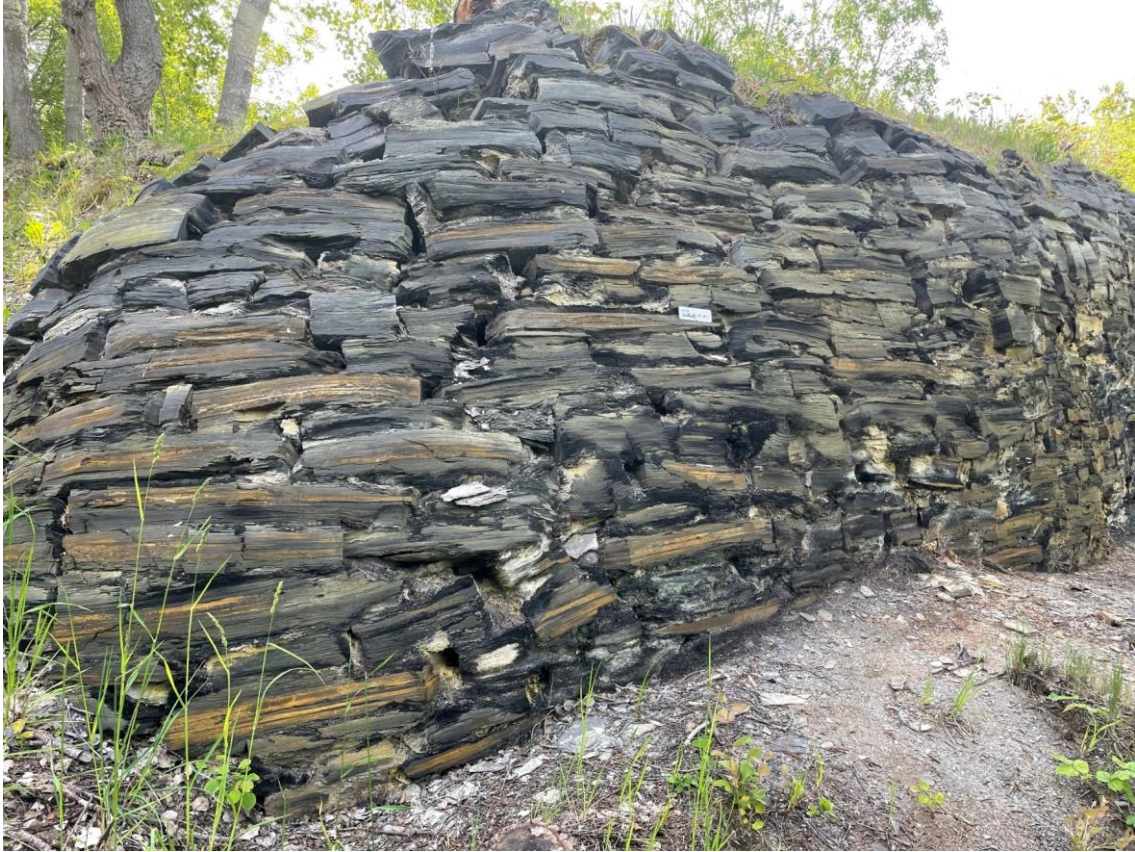
Figure 28. Black shale blocks used to build kilns. Photo: Anna Ladenberger.
