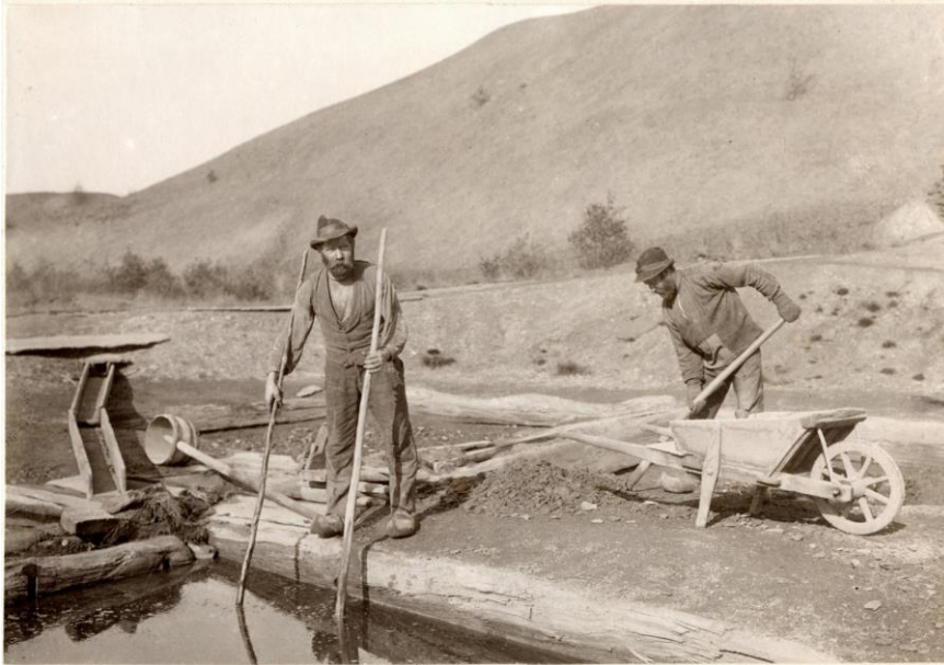
Figure 24. Leaching pools in the alum factory at Andrarum, 1910. Waste heaps with burnt shale can be seen behind the workers. Photo: Alfred B. Nilsson (Tekniska Museet).
