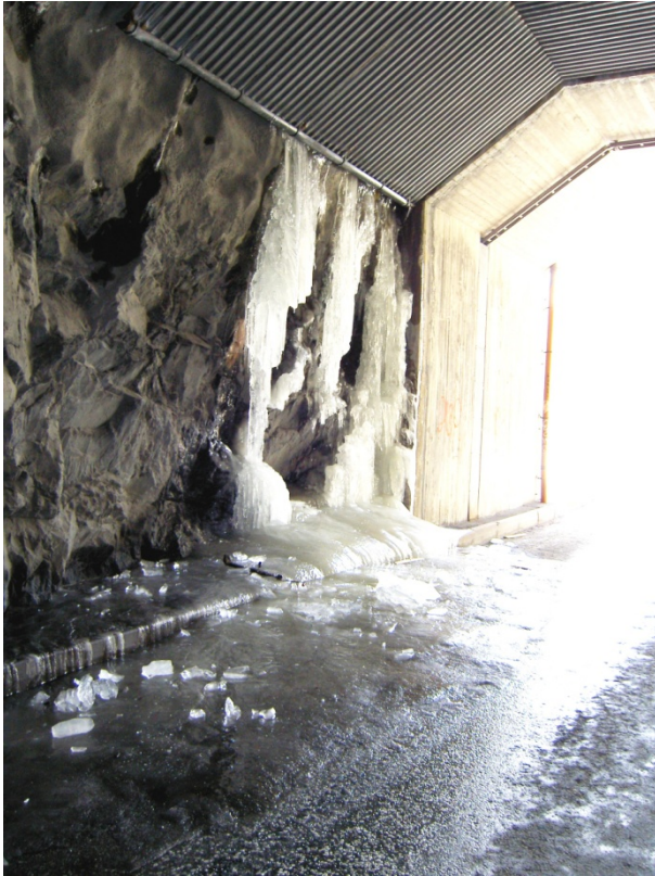
Figure 9. Ice formation in the Finnberg tunnel before remedial measures.
