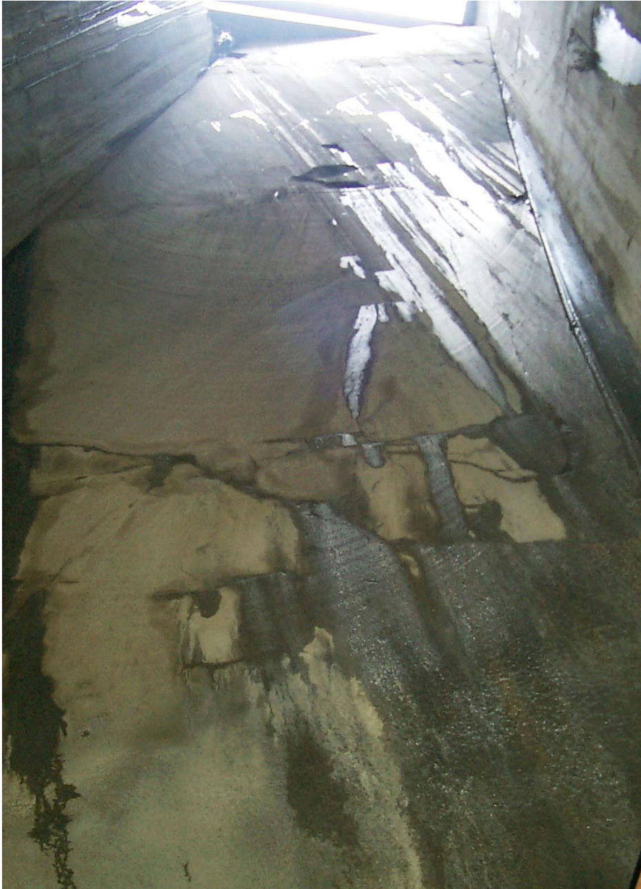
Figure 12. Wire sawing is used more often to prevent vibrations propagating and adversely affecting existing buildings.
