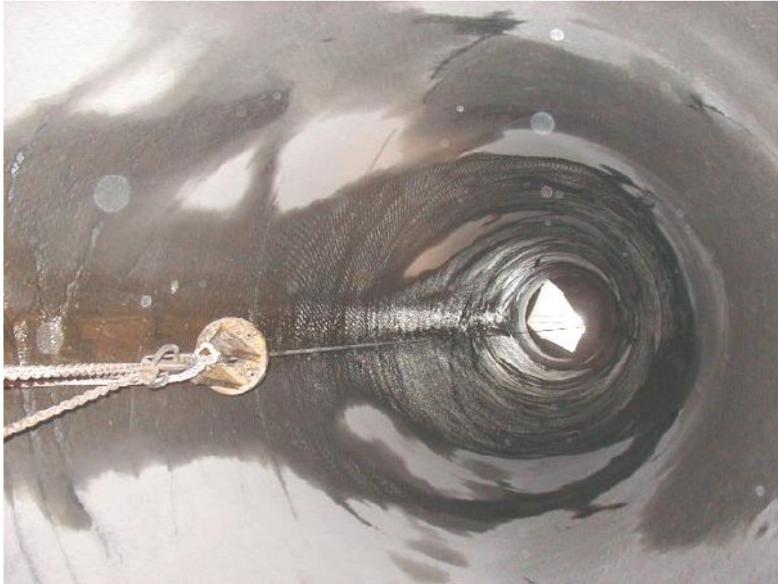
Figure 13. Raise-bored ventilation shaft.
