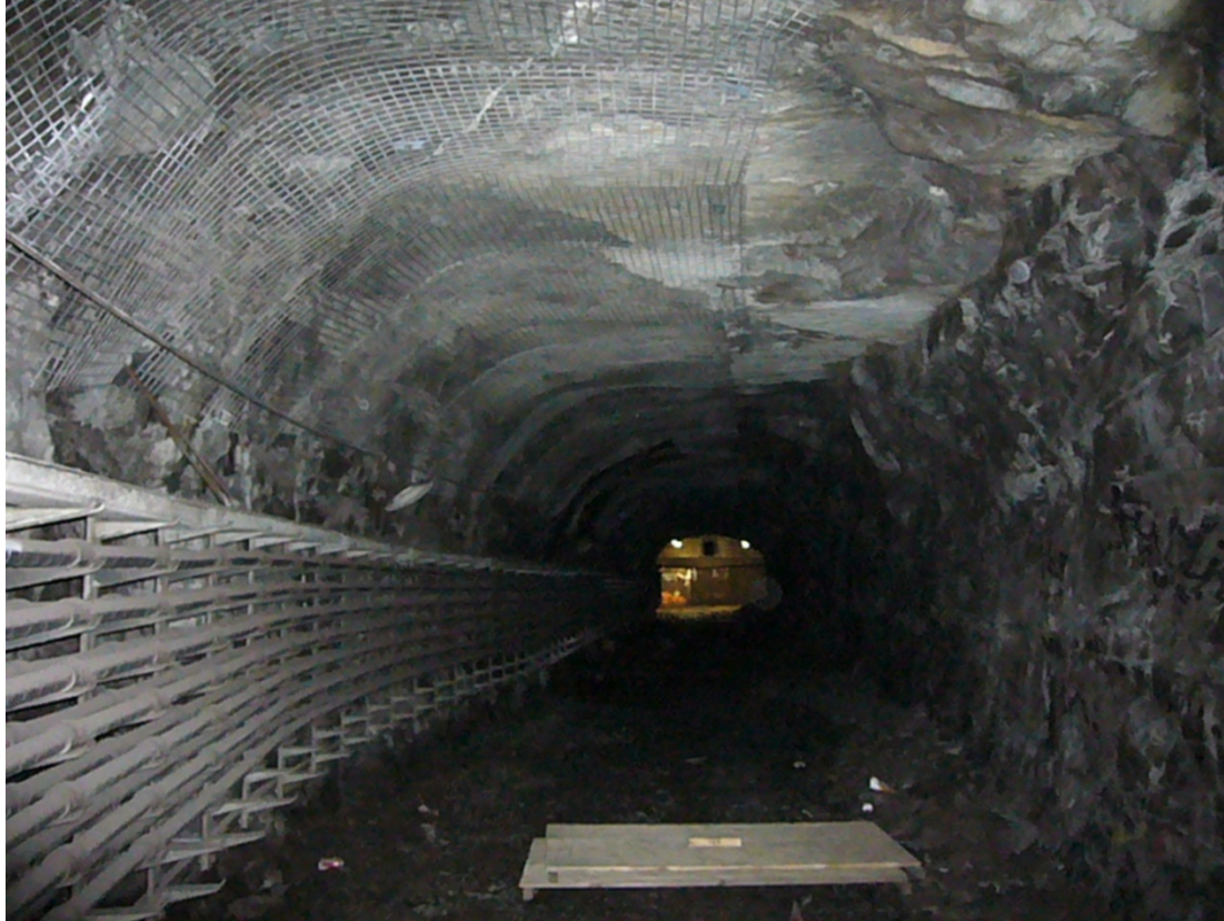
Figure 2. Ventilation tunnel at Hälsingehöjden. Failing of thin rock slabs and even evidence of rock bursts behind a reinforcement grid in the roof.
