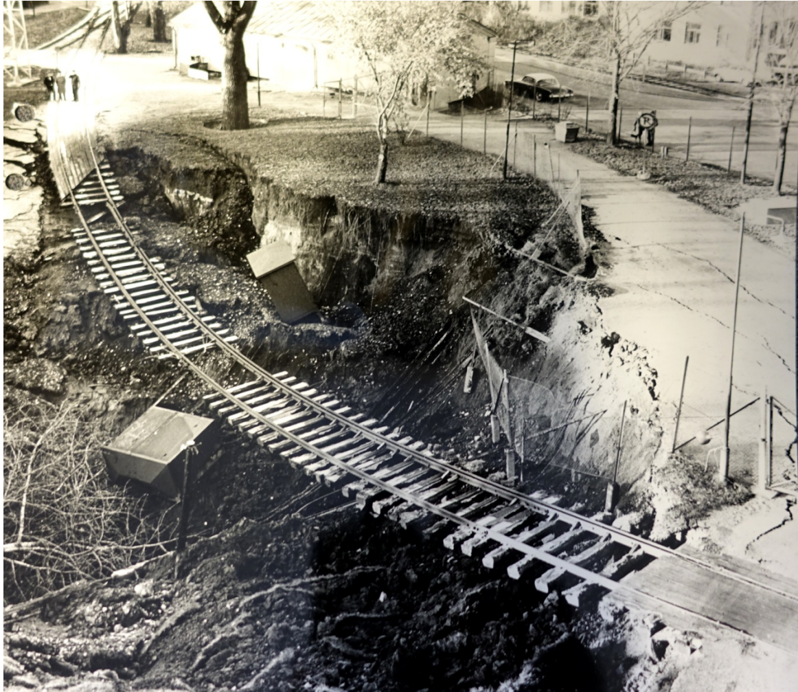
Figure 4. The tunnel collapse that occurred in 1965 at Mårtensdal, Södra Hammarbyhamnen.
