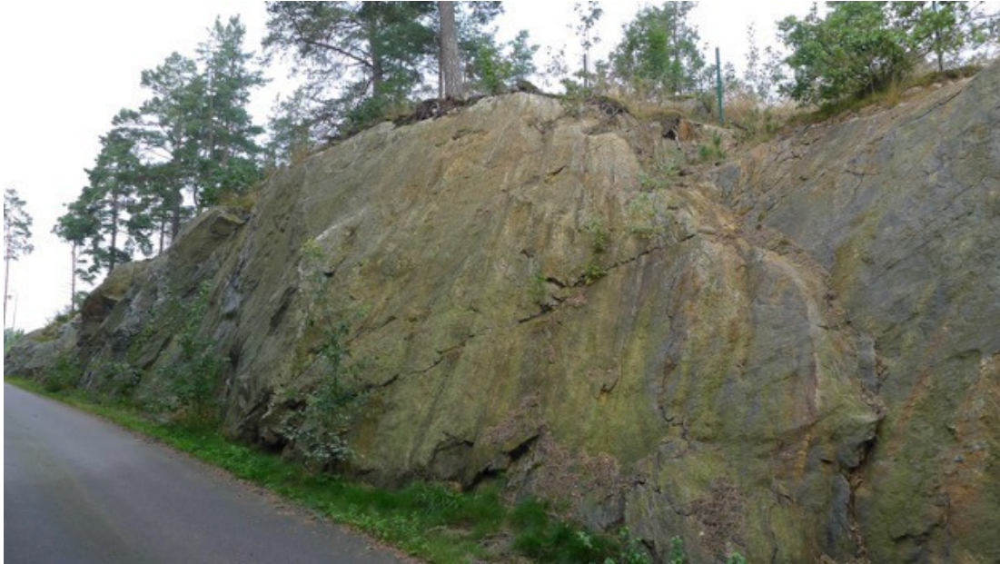
Figure 6. Rock cutting at Smista Allé. The rock cutting is about 3 m high. Due to sliding along a foliation surface, the slope of the face has become flatter than the drilled contour design, which was vertical. The limited face height resulted in a manageable outcome, and the slope is now stable as it now is compatible with the existing rock structure. Photo: Lars Bergkvist, Golder.
