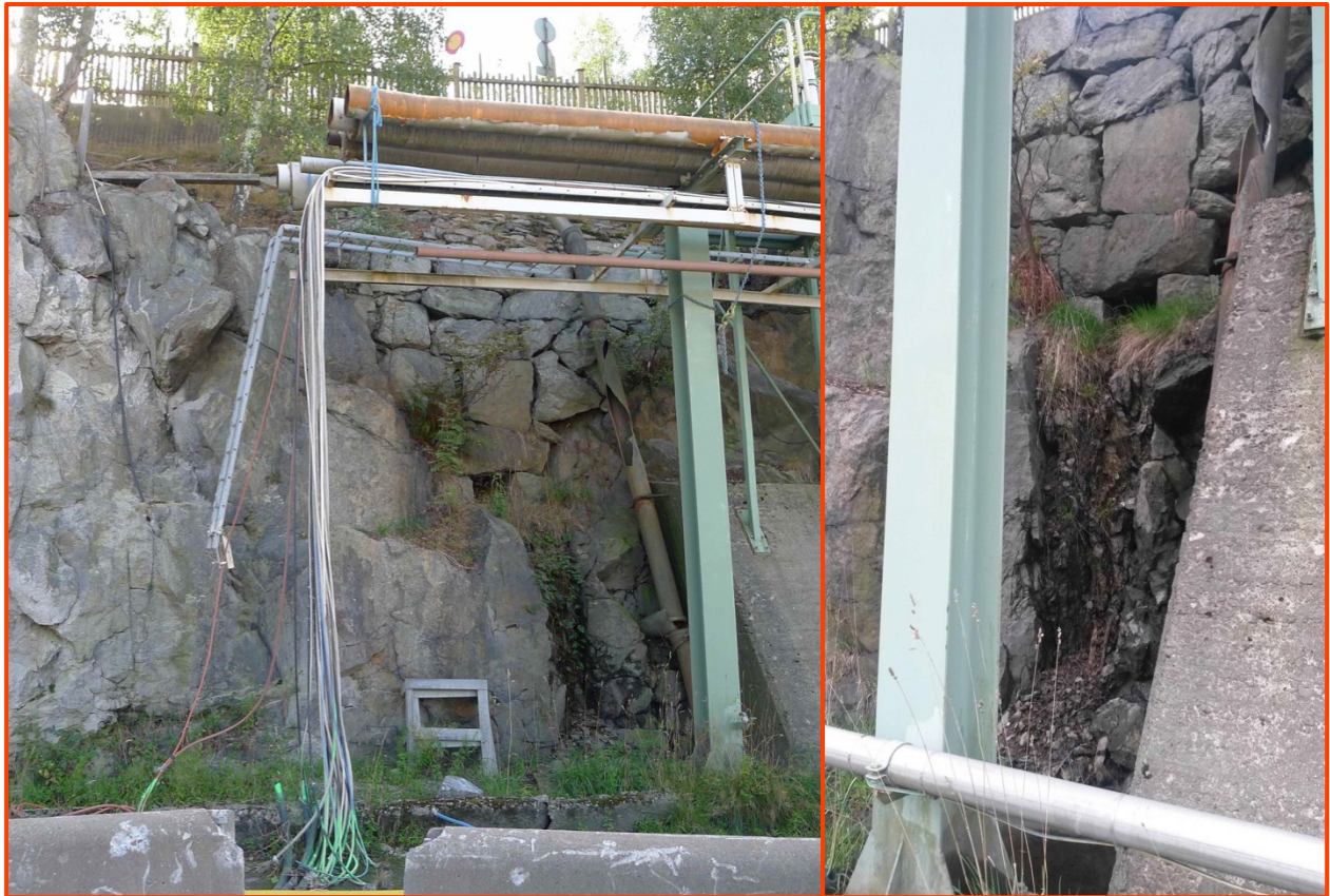
Figure 12. Hjorthagen. Fracture zone indicated on the Construction Geology Map. Overview and close-up. Photo: Sofie Eskilander, Golder.
