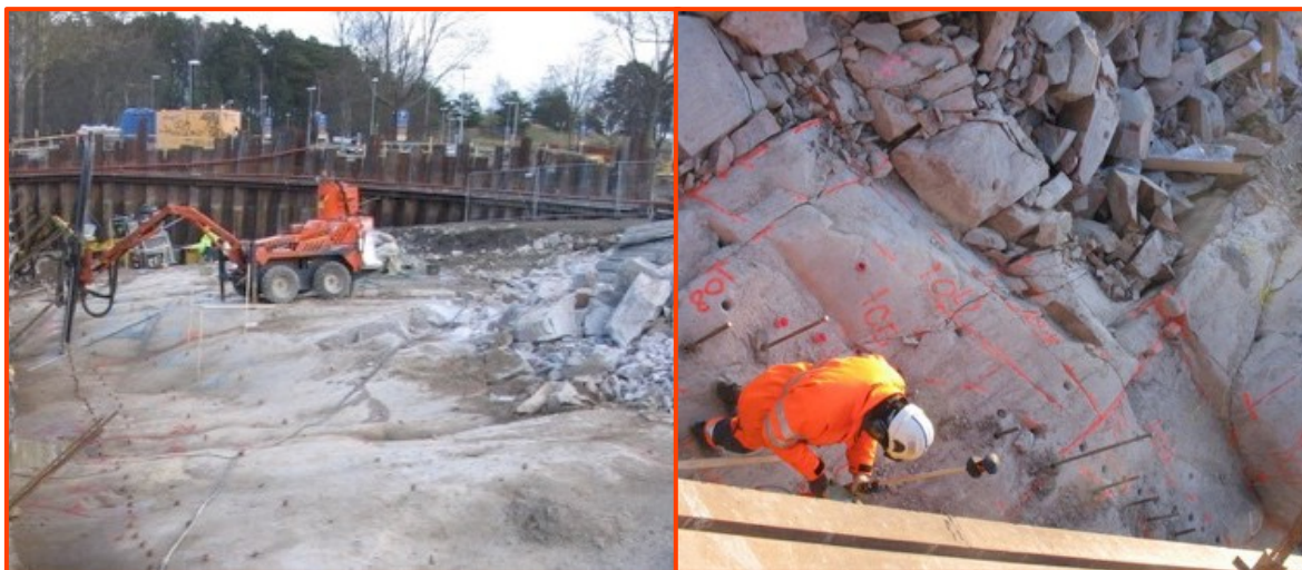
Figure 1. Täby. Left: drilling of contour holes next to a sheet pile wall. Right: in the upper half of the photo, bedrock unintentionally shattered by blasting gases from a round 4m away can be seen. Photo: Lars M Hansen, Golder.
