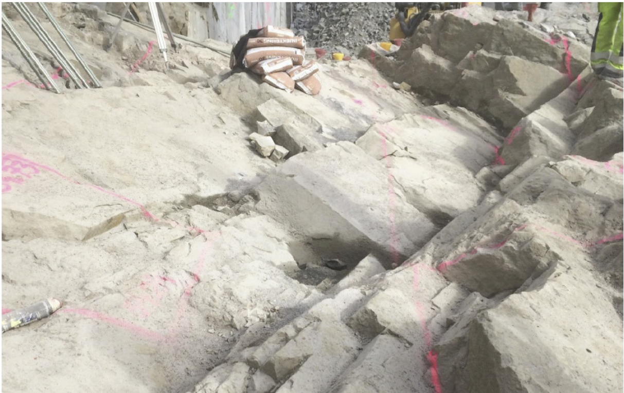
Figure 20. Southerly dipping fractures at Södersjukhuset. Photo: Lars Bergkvist, Golder.
