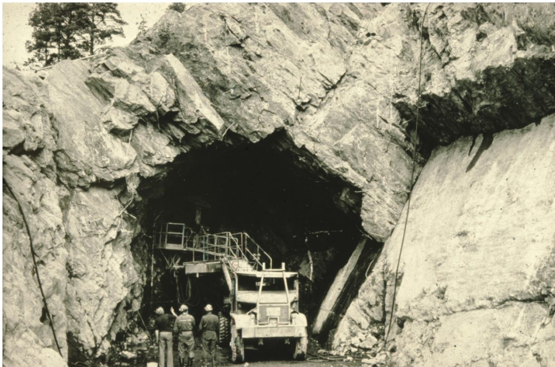
Moderately dipping fractures at the tunnel portal for a de-icing facility in Älvsjö.
