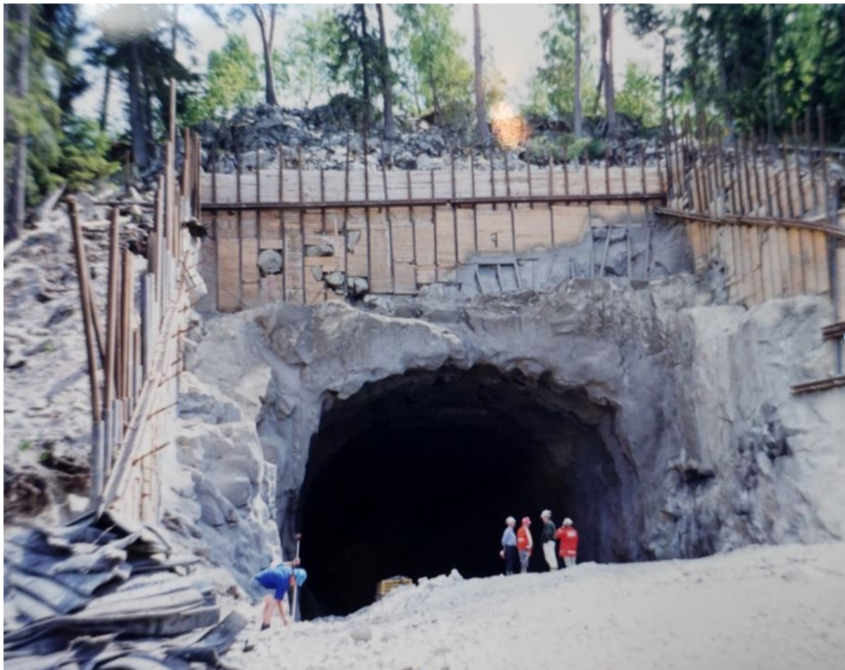
Figure 1. Railway tunnel south of Kungsängen. Blocky till on top of an irregular bedrock surface.
