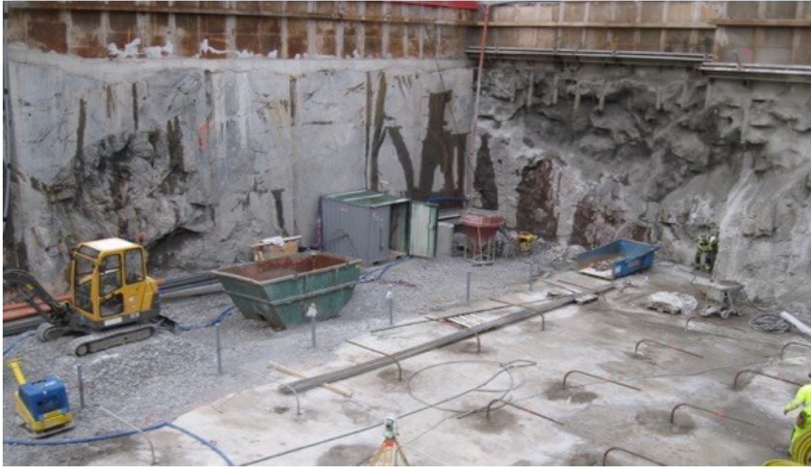
Figure 35. Excavation with drilled pile wall consisting of casing and welded plate, where the rock wall to the left has been cut with a wire saw and blasted to the right. Below the foot (dark area to the right of the middle, where the lower end of the feed tube hangs) blocks have slipped out, a slip of the same type as shown in Figure 8. Photo Mikael Creütz, Golder.
