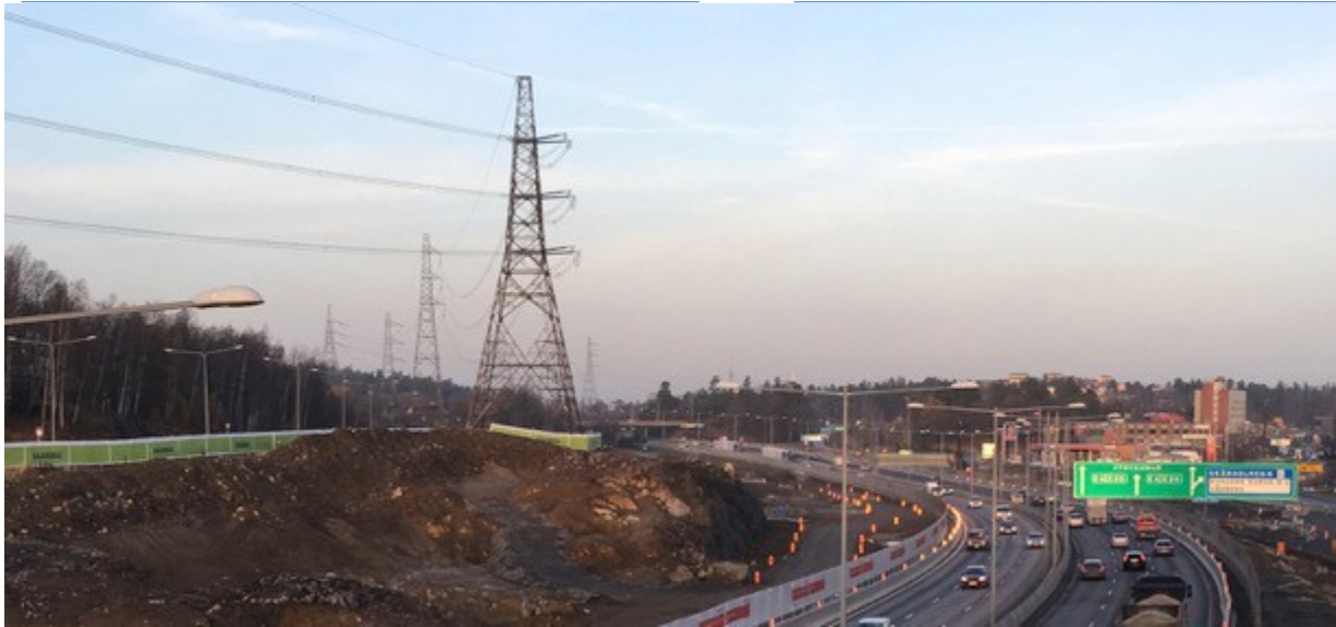
Figure 11. Power cable mast founded on rock. Along the Skärholm road and along the E4 / E20 there are planar structures with unfavourable orientations for stability (see Figure 8) and sliding of the same dimension as shown in Figure 7 can cause major damage. Therefore, rock excavation is carried out very carefully, and continuous measurements are made of the foundations to determine whether movement occurs. Photo: Lars M Hansen.
