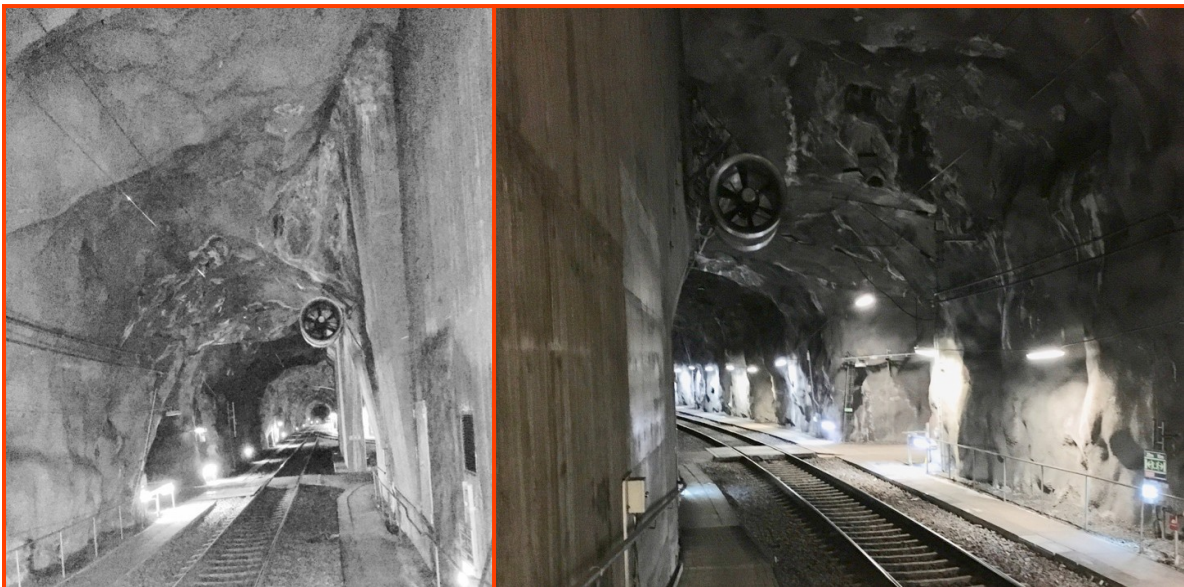
Figure 28. Arlandabanan, southern end of Arlanda N station (terminal 5). Here there was a movement, -heave in the roof, in connection with blasting. The crack that occurred between the rock pillar and the overlying rock mass cannot be seen in the picture as it is covered with shotcrete and the cast concrete pillar. Photo: Lars M Hansen.
