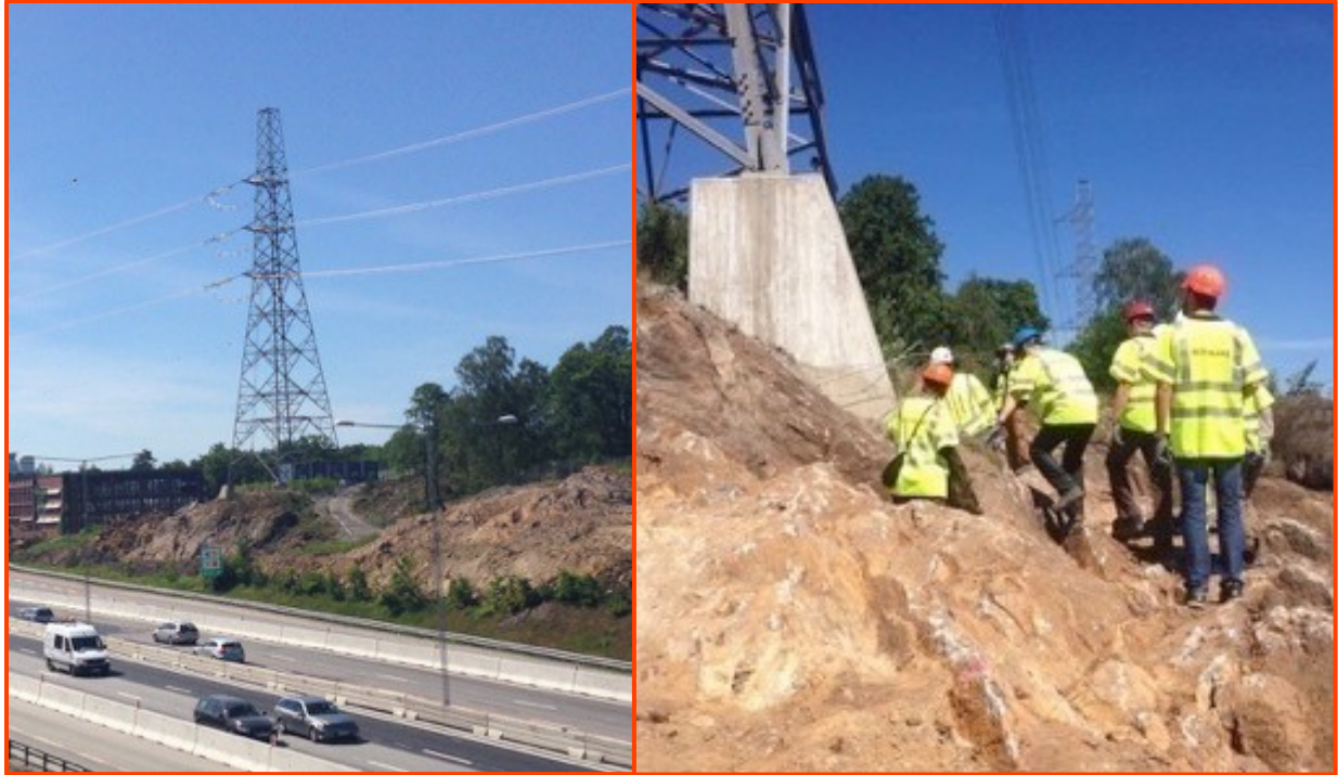
Figure 9. Power line mast near to a road to be widened. The rock mass consists of sedimentary gneiss of less good quality and with weathered sections. Photo: Lars M Hansen.
