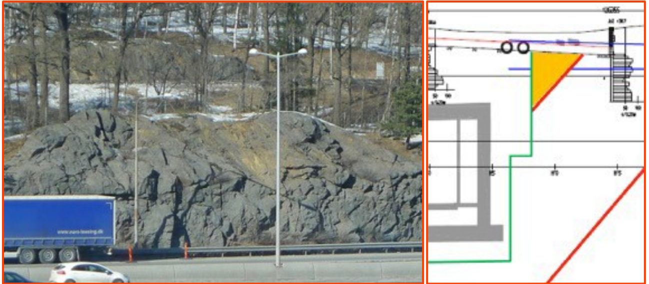
Figure 8. Rock cutting at E4 / E20 at Kungens Kurva. The rock cutting is about 6 m high. The contour holes have been drilled vertically, but due to rock slides, the upper slope profile has become flatter. The exposure of the failure plane high on the slope limited the slide volume. The lower red line, in the right figure, indicates a structure that is far enough from the shaft to form support for the rock mass. Photo: Lars M Hansen.
