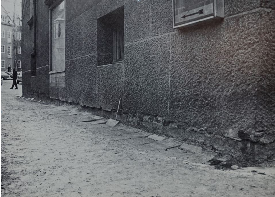
Figure 6. Karlaplan area 1964. Subsidence of the street adjacent to a building supported on wooden piles.
