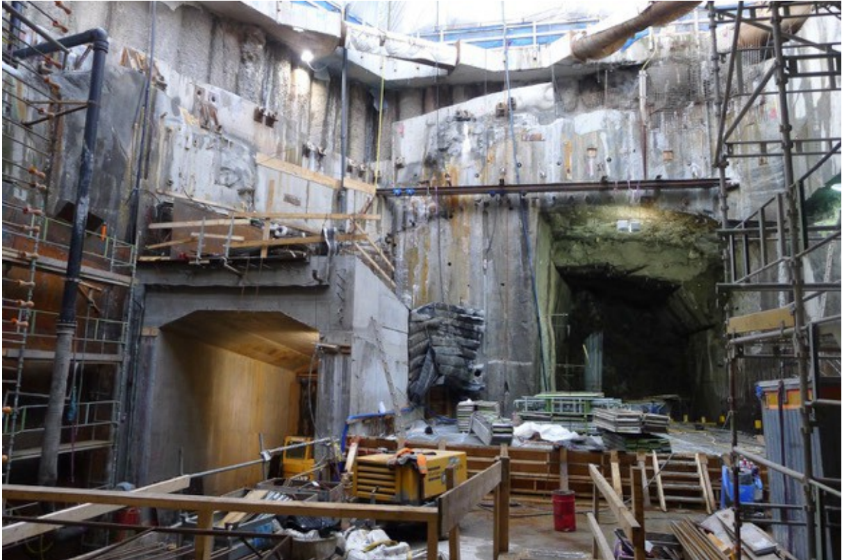
Figure 14. Riddarholmen. Excavation in bedrock, isolated from Riddarfjärden's water with the help of secant pile walls (concrete diaphragm/concrete bored pile wall) which are seen at the top of the road in the photo. Careful rock excavation is being performed by wire sawing when the rock cover is small. A depression in the rock surface above the concrete tunnel has been filled with concrete. The depression is due to an approximately 0,5 m wide fracture zone (Figure 13), which is oriented NW with a dip to the SW. Photo: Anja Olsson, Golder.
