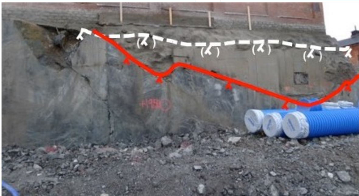
Figure 32. The figure shows the interpreted (white) bedrock profile based on probes and the real (red) bedrock profile, as well as the supporting walls that needed to be built. Photo: Edward Runslätt, Golder.
