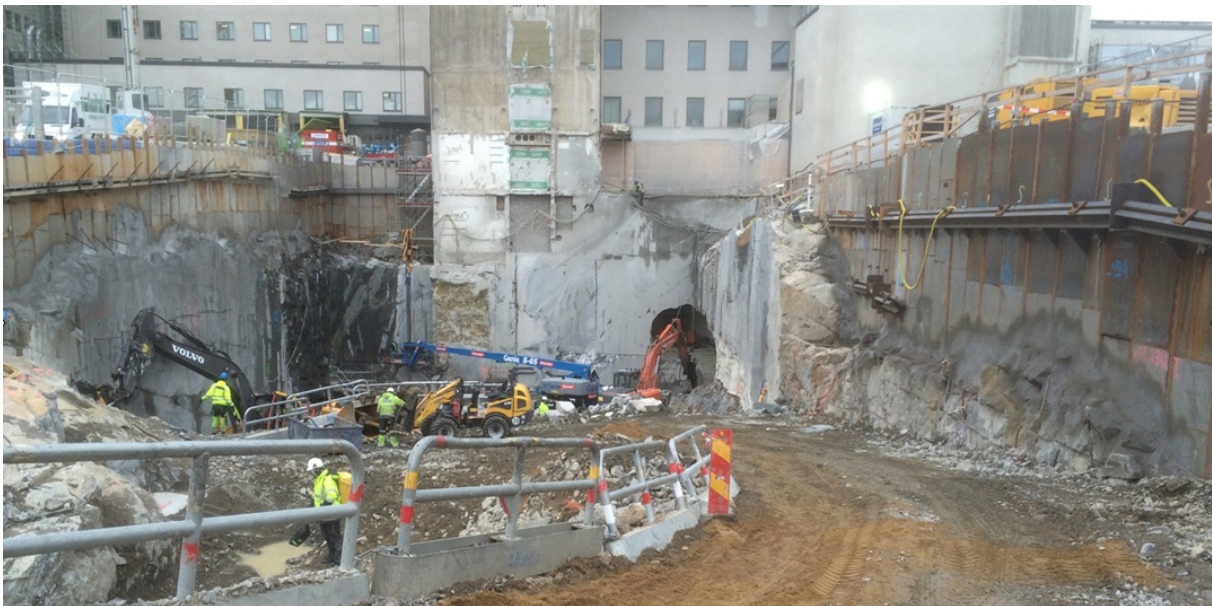
Figure 15. Södersjukhuset. Wire sawn 10 m high rock walls next to existing buildings. Prior to sawing, rock reinforcement has been installed in the form of a long bolt set from the top of the planned cut. Photo: Jörgen Theander, Golder.
