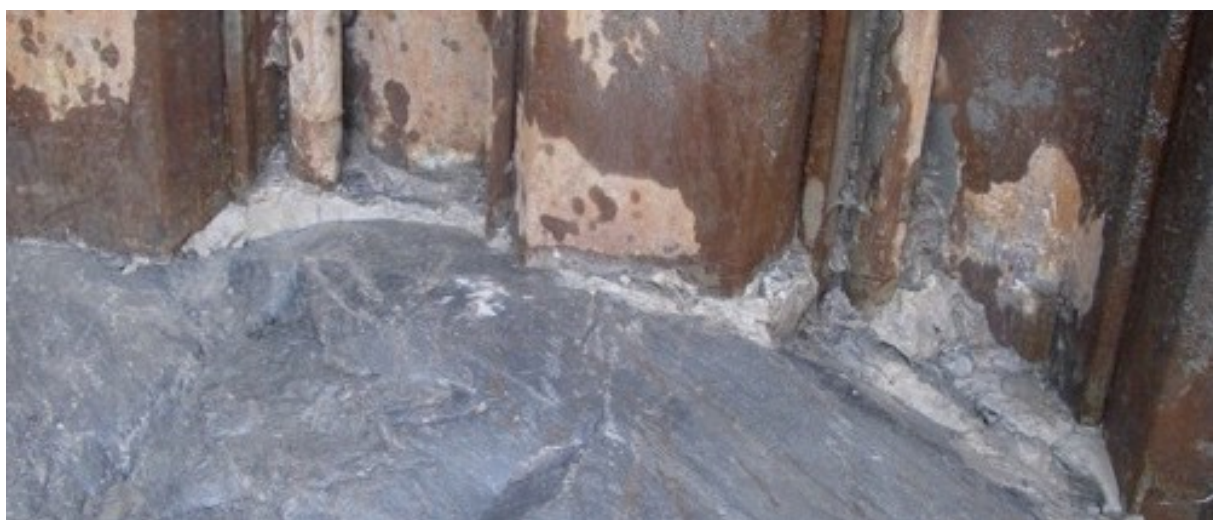
Figure 34. Grout at the contact between the sheet pile wall and the bedrock. Photo Mikael Creütz, Golder.
