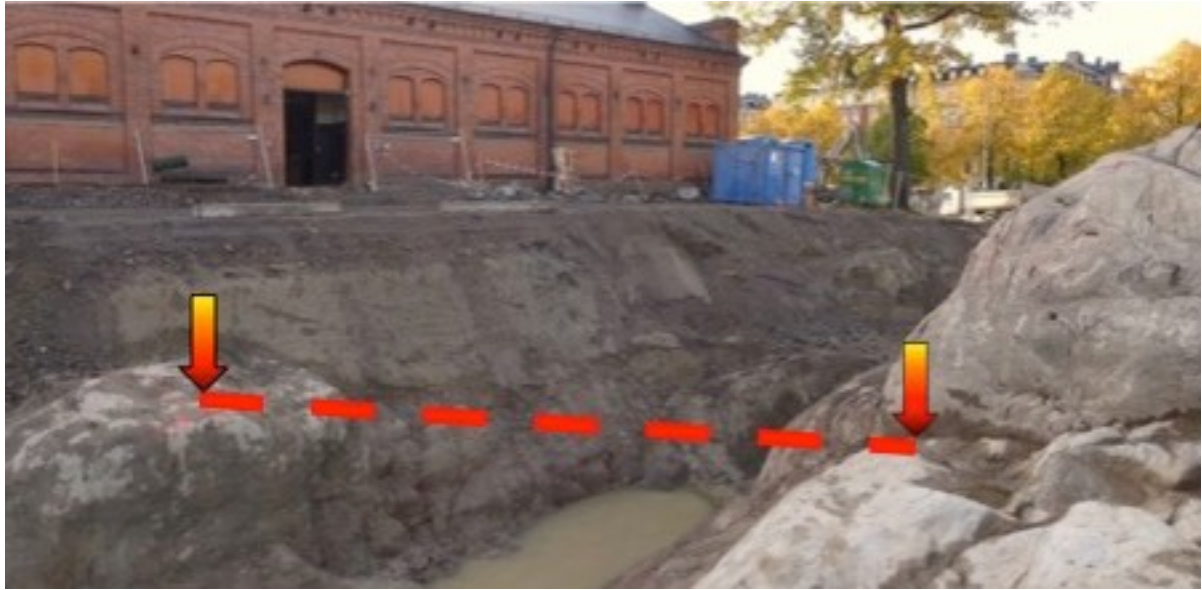
Figure 31. Example of how bedrock probing can give rise to a misleading interpretation. When probing was performed at the arrows (cc about 10 m) the depression was missed. Photo: Edward Runslätt, Golder.
