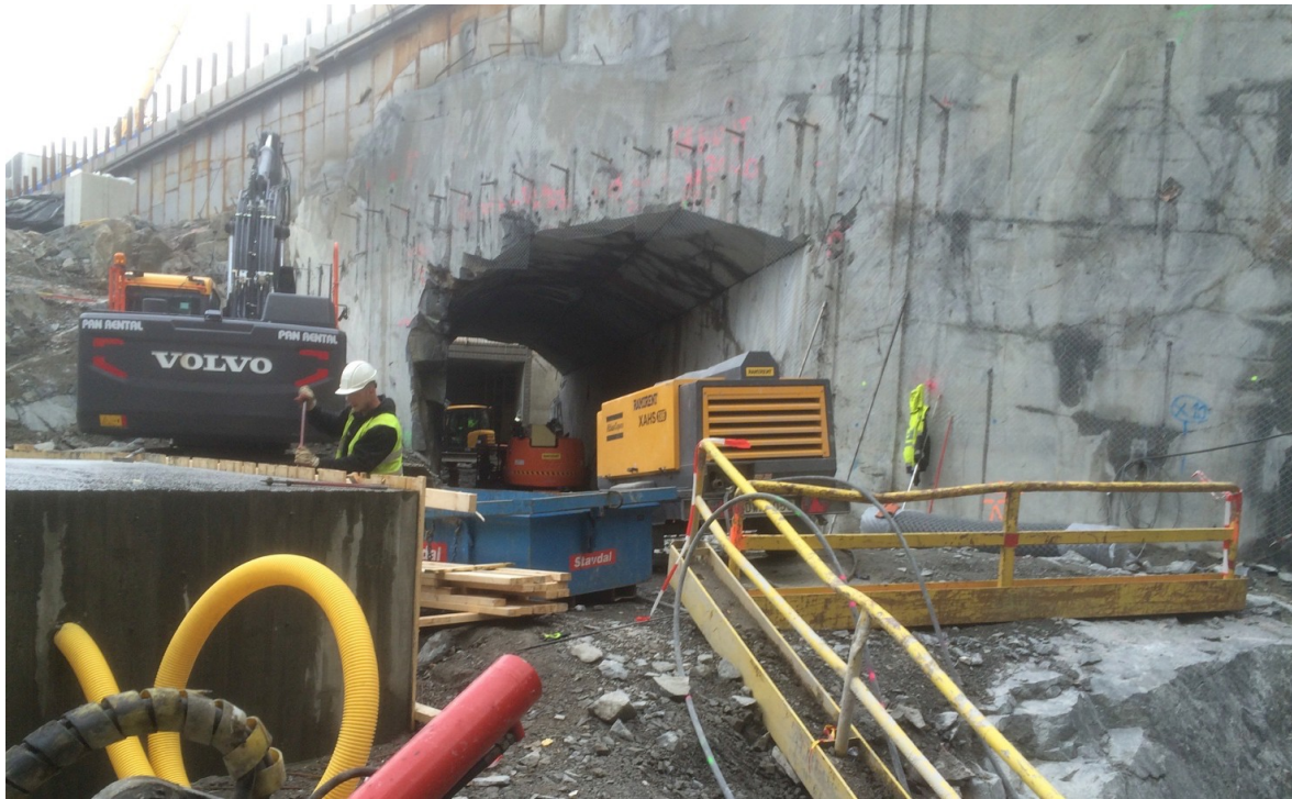
Figure 16. Tunnel with limited rock cover. The tunnel is reinforced above the planned roof line before rock excavation and the contour is wire sawn to prevent explosive gases penetrating rock fractures to crack and causing an excessive damage zone in the rock around the tunnel. Photo: Jörgen Theander, Golder.
