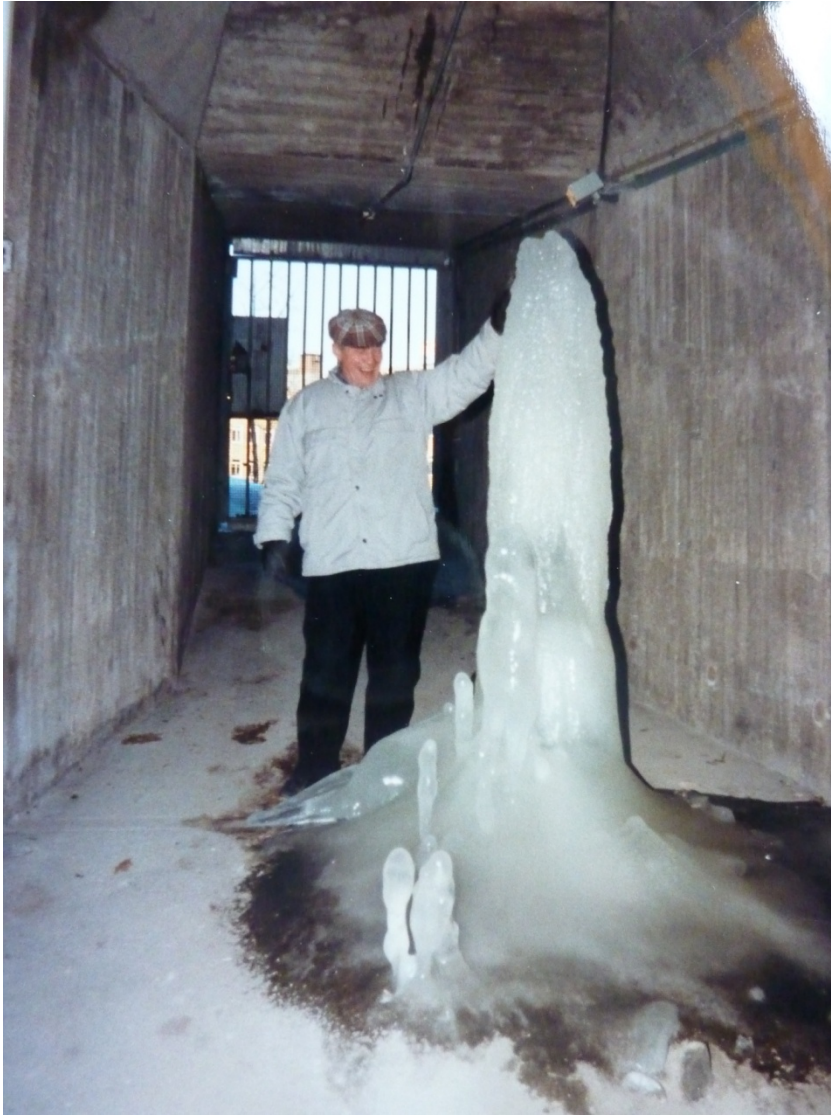
Figure 8. Ice build up in a tunnel.
