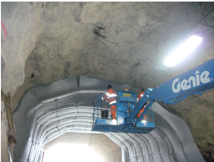
Figure 10. Sheets of extruded polyethylene being installed in the roof and walls at the portal and for a distance into the Finnberg tunnel.
