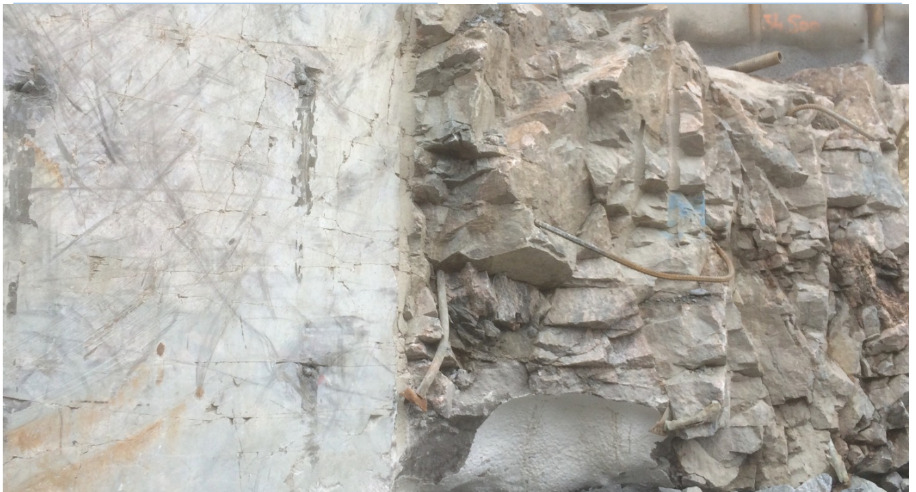
Figure 17. Comparison of a sawn and blasted rock mass, where the sawn surface also needs to be reinforced. A sawn surface can be treacherous and attention is required since the fractures do not appear as clearly. Photo: Jörgen Theander, Golder.
