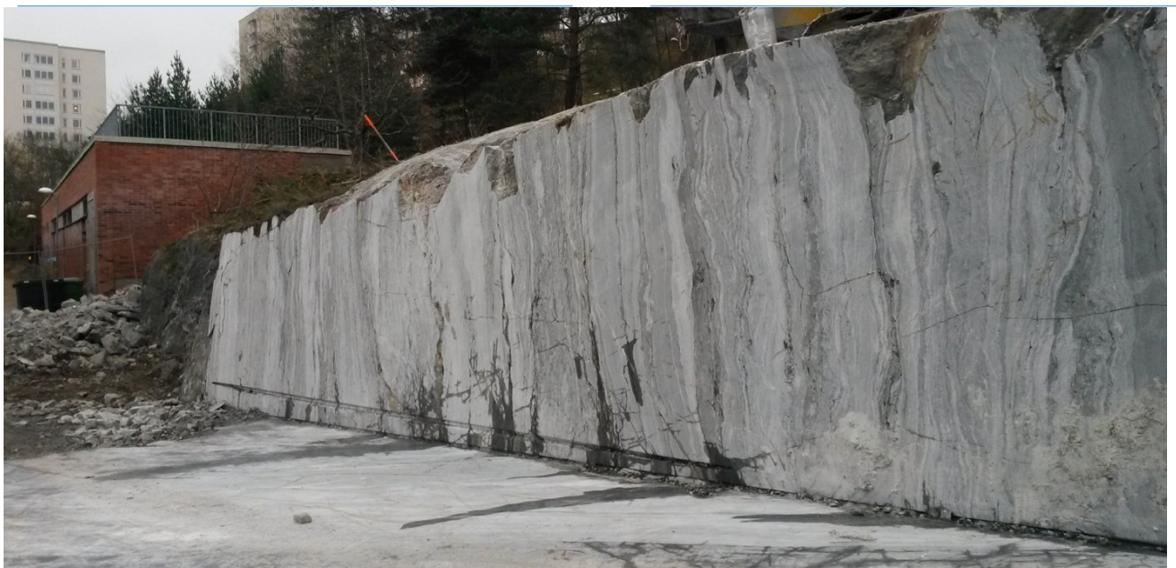
Figure 3. Liljeholmen. Wire sawn rock cut with irregular stress relief joints and steeply dipping gneissic banding/foliation. The rock cut lies above an existing tunnel; both horizontal and vertical wire sawing has been performed to comply with vibration restrictions due to a nearby elevator shaft. Photo: Anja Olsson, Golder.
