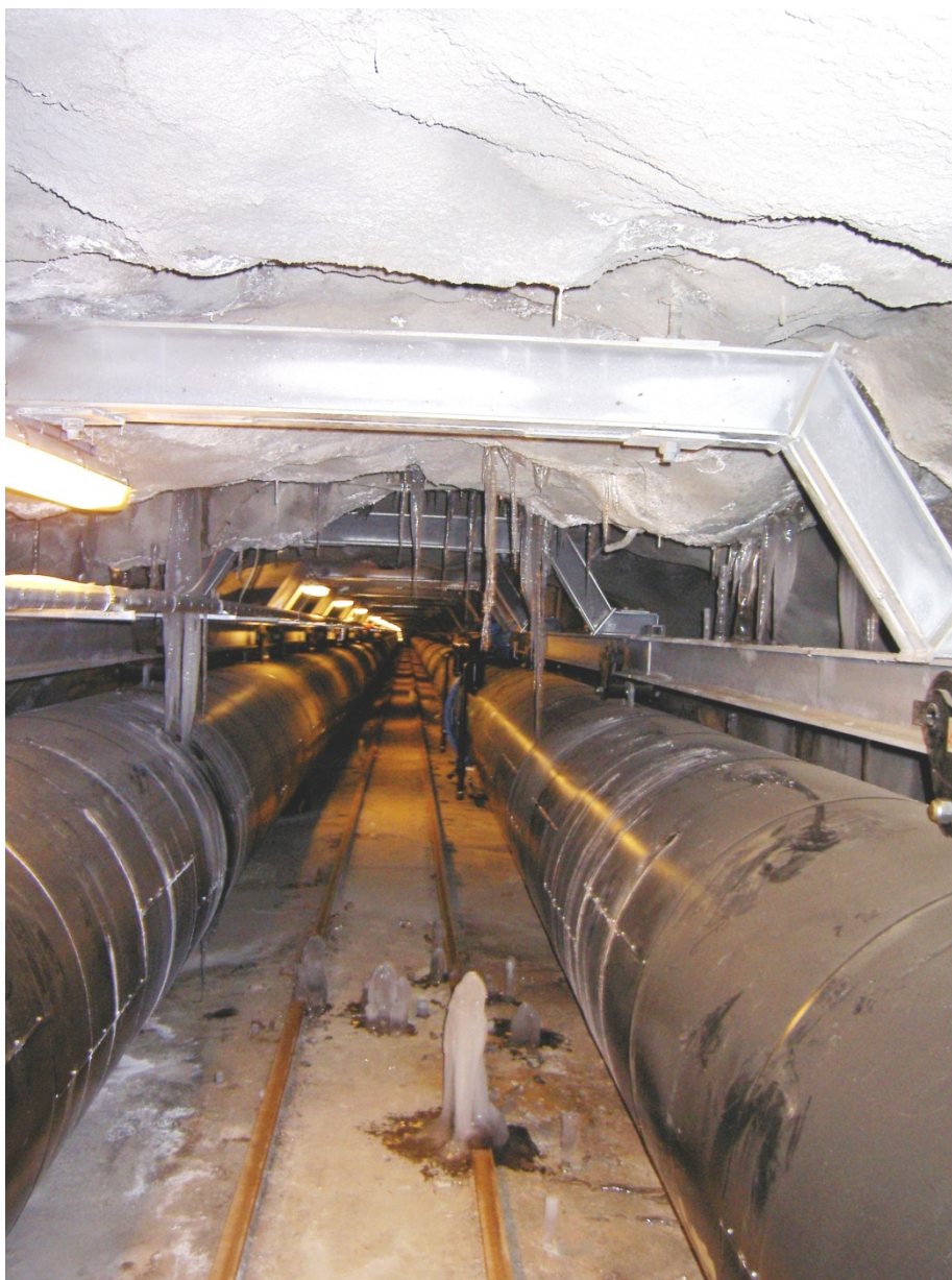
Figure 14. Heavy pipes suspended from the tunnel roof. Load testing was necessary to ensure the capacity of the rock anchors.
