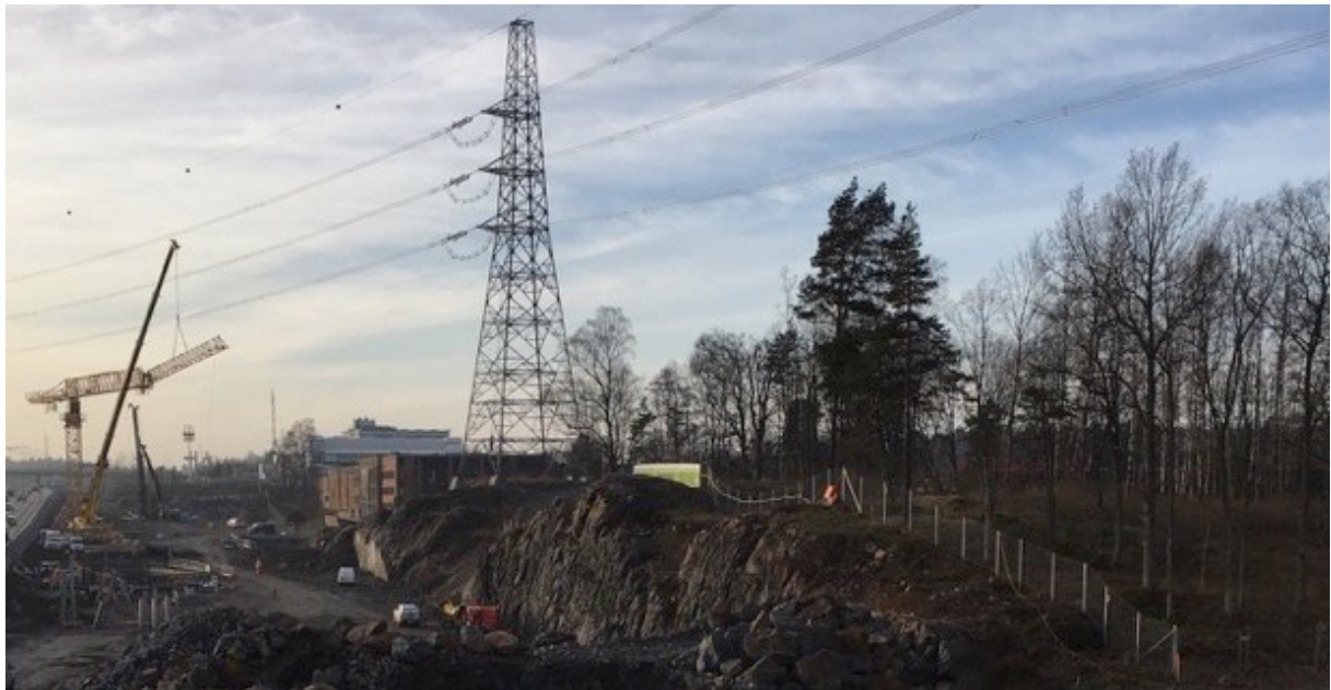
Figure 10. Same power line as in Figure 9. The planned cut was moved a few metres from the initial position and was sawn in three sections. One of the sawn sections is clearly visible to the left of and below the mast. Photo: Lars M Hansen.
